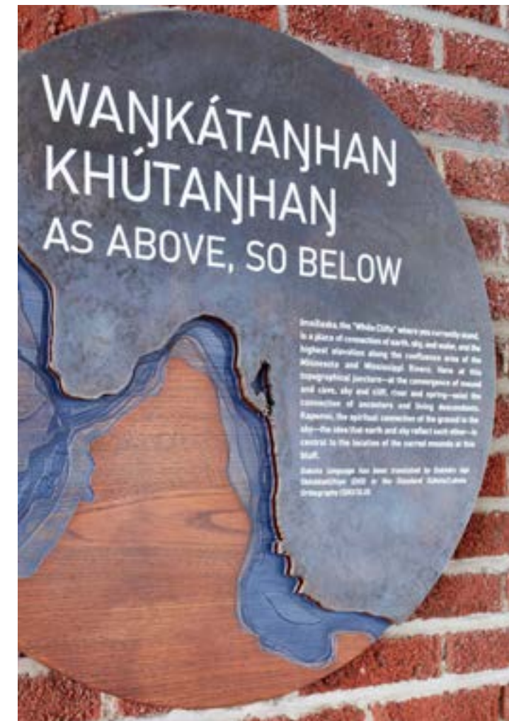
Blackened steel with chemical treated wash and etched letters painted white
