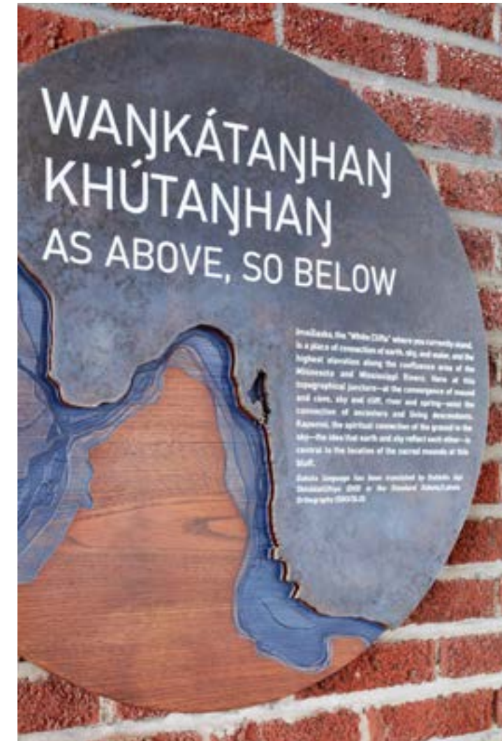
Blackened steel with chemical treated wash and etched letters painted white
