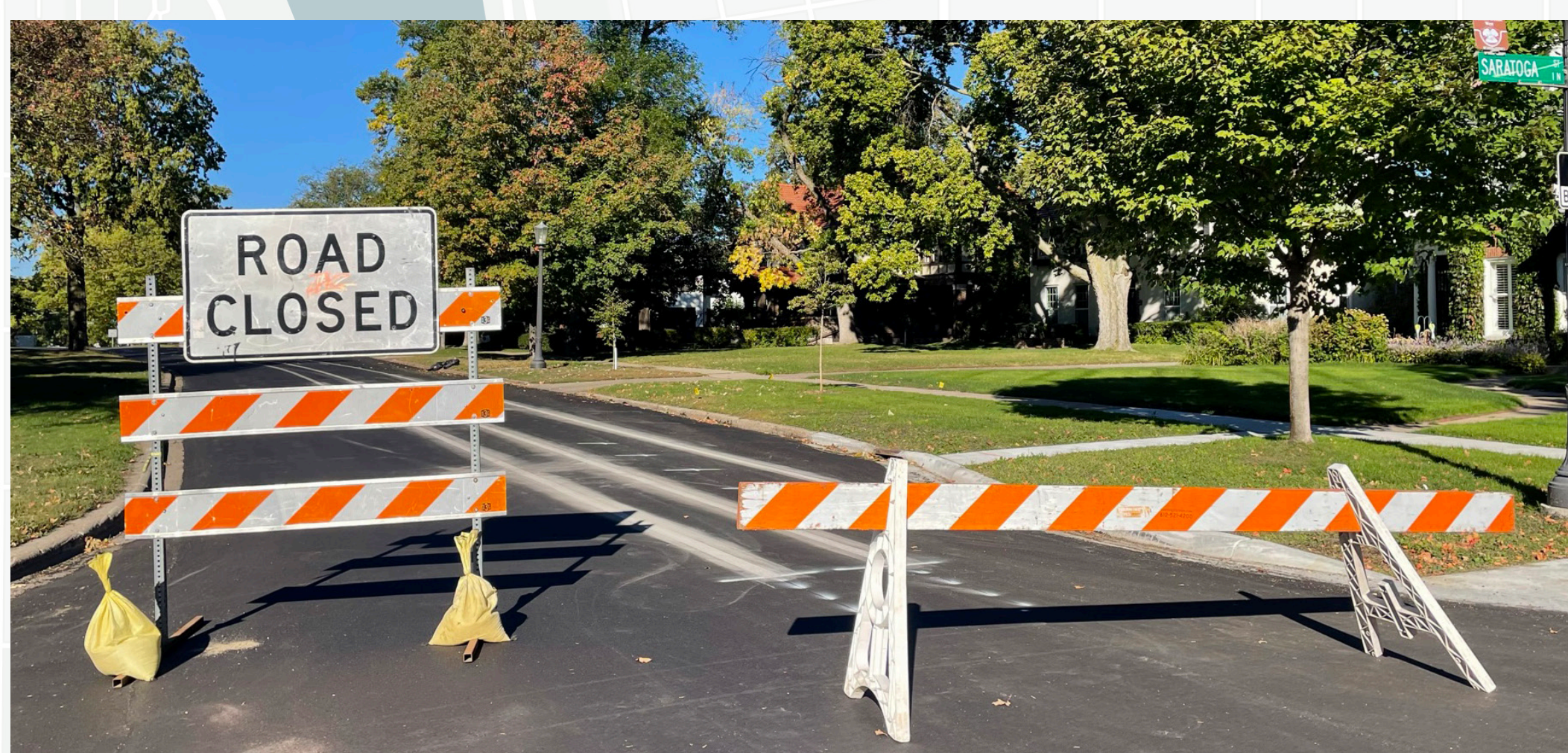
2022 mill & overlay and crossing improvements on Summit Avenue
