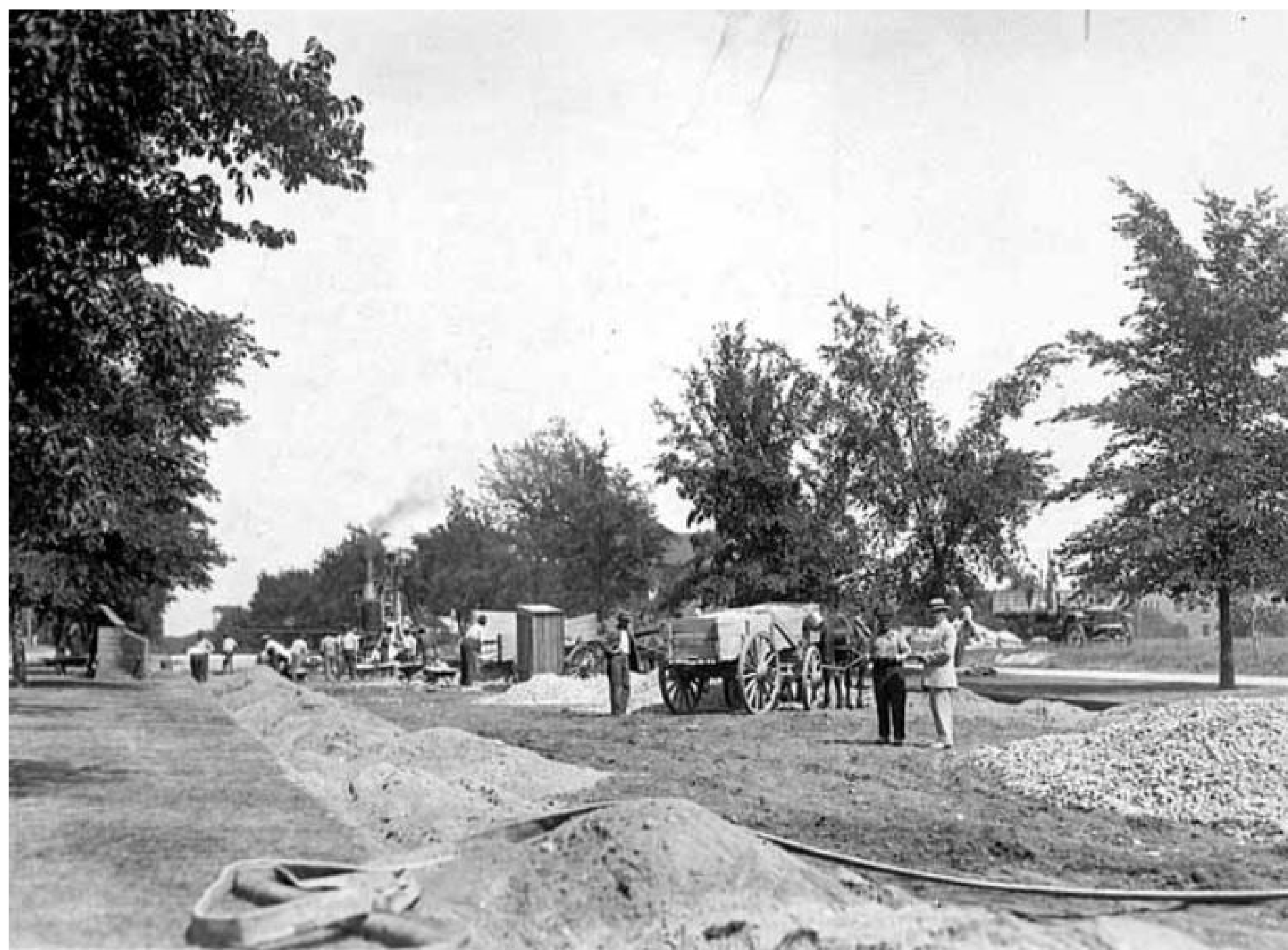
Roadway construction near Summit Avenue and Grotto, 1915 | Credit: Minnesota Historical Society
