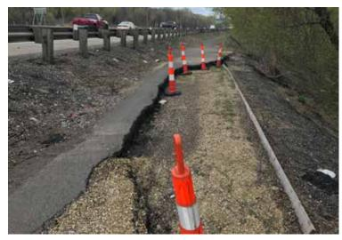
Segment 1 slope failure along southbound Hwy 61.
