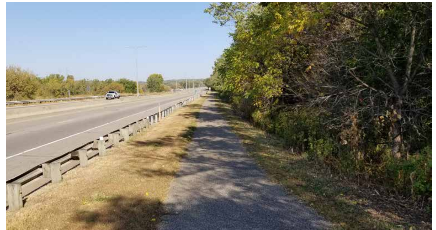
Segment 4 looking north. Notice existing 8'-0" trail.
